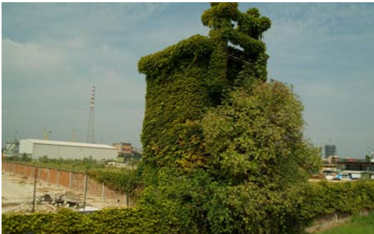
Former distribution sub-station
