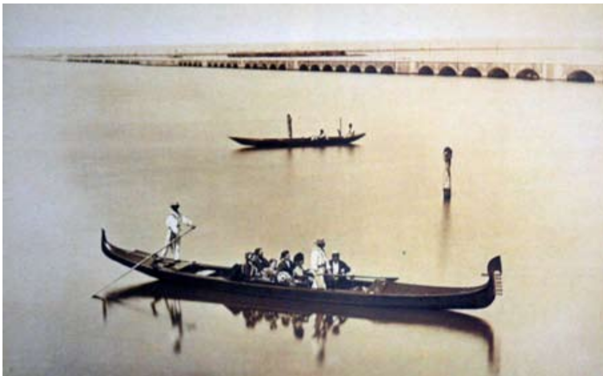
The old and the new connection to Venice
