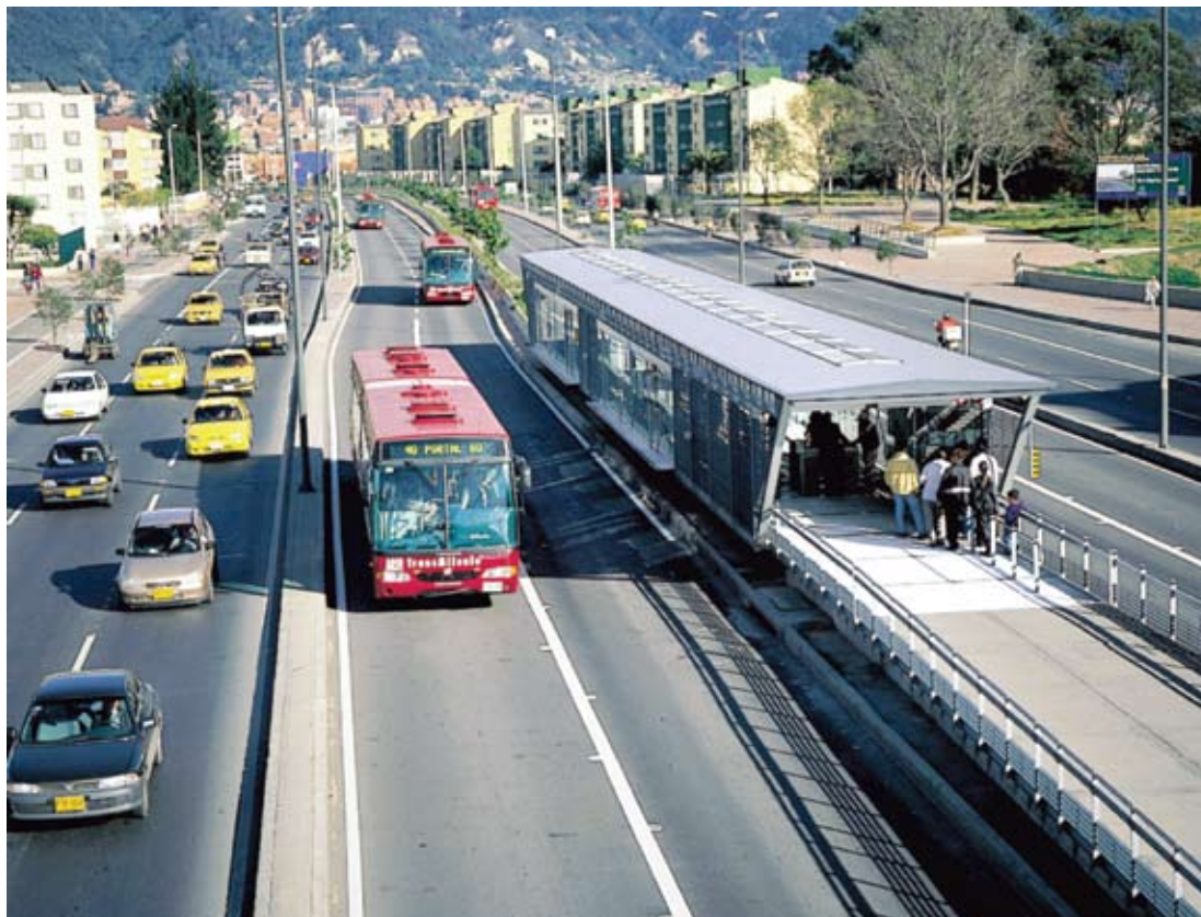
Figure 9: The Bogota TransMilenio is derived from the pioneering Curitiba Bus Rapid Transit (BRT) network that started in 1976 which has proven its mass transit capacity while providing for enhanced safety and security through its staffed stations. BRT achieves very high commercial speeds, as it is given a total right-of-way and all ticketing takes place at stations. Note the possibility of express buses to pass all-stops buses. In narrower roads and urban streets, space can be saved by using guided buses (e.g. through an optical guidance system)
